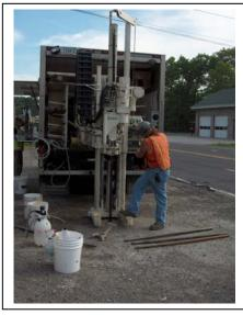
In June, **piezometers** were installed in the Area of Investigation. A piezometer is a small well (usually about 1 inch in diameter) that is used to measure the depth below the ground surface that groundwater is first encountered (called the "water table" or "water level"). Water levels will be measured each season during the Field Investigation.
