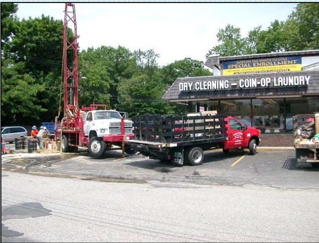
**Photograph 1: Drill Rig Installing Monitoring Well**
